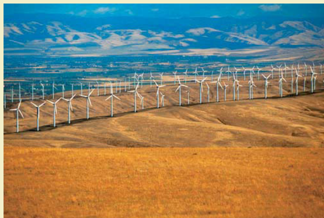
This State Line Wind Project along the Oregon-Washington border uses approximately 399 wind turbines to create enough electricity to power some 70,000 households.
